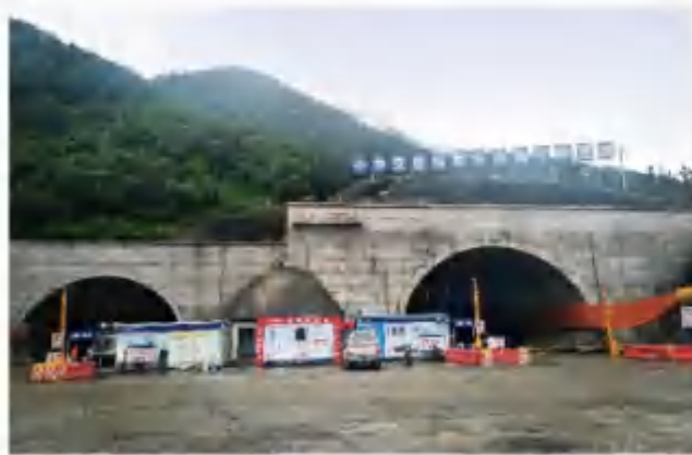
广东省开春高速公路坳仔岭隧道超前地质预报与监控量测 Advance geological prediction and monitoring measurement of aoziling tunnel of Kaichun Expressway in Guangdong Province
