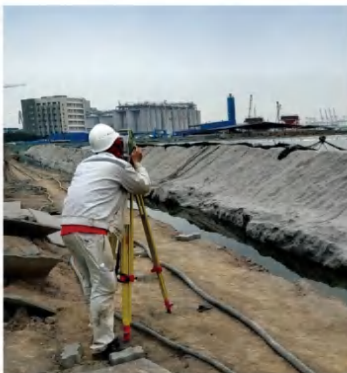
广州港南沙港区粮食及通用码头扩建工程 真空预压地基处理第三方监测 Third party monitoring of vacuum preloading foundation treatment for grain and general wharf expansion project of Nansha port area of Guangzhou Port
