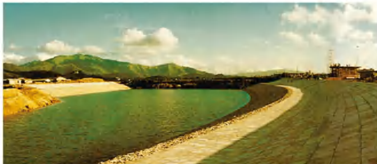
深圳河一期工程边坡施工监测 Construction monitoring of slope for the first phase engineering of Shenzhen River
