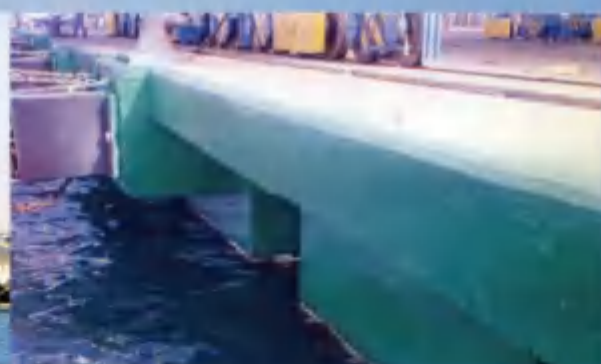
苏丹港码头钢管桩铝合金牺牲阳极保护和钢筋混凝土梁板涂层防腐设计 Design of aluminum alloy sacrificial anode for steel pipe piles and anticorrosion coating for reinforced concrete beams and slabs of Port Sudan
