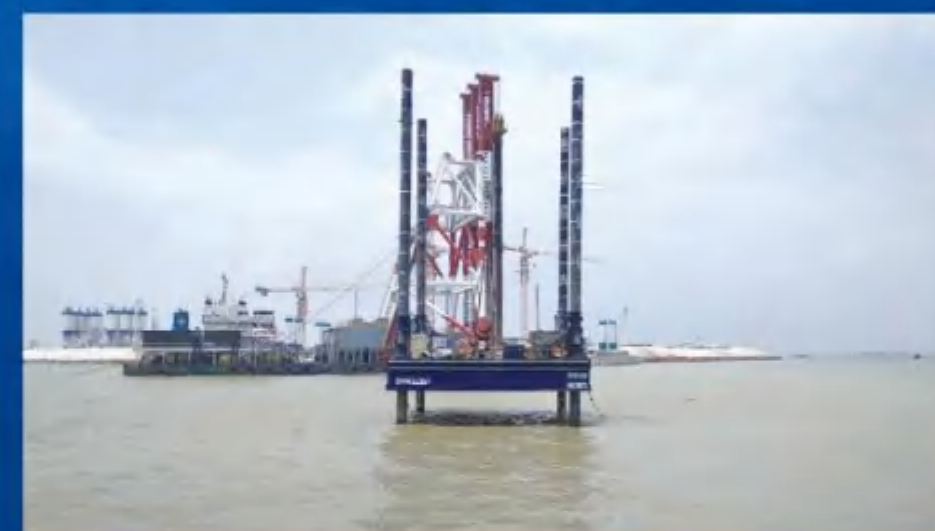
深圳至中山跨江通道主体工程（S09 标）DCM 检测 Testig of DCM for Main Project of Cross-River Passage from Shenzhen to Zhongshan ( Bid S09 )
