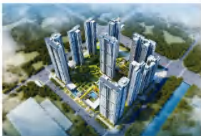
中交邮轮母港二号地块（中交蓝色海湾）基坑监测 Monitoring of building excavation for Plot 2 of Cruise home port of CCCC
