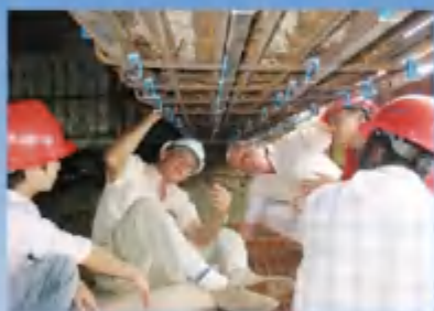
肯尼亚蒙巴萨港KIPVU桥外加电流防腐设计 Design of impressed electric current anticorrosion protection for Kipevu Bridge in Port of Mombasa, Kenya
