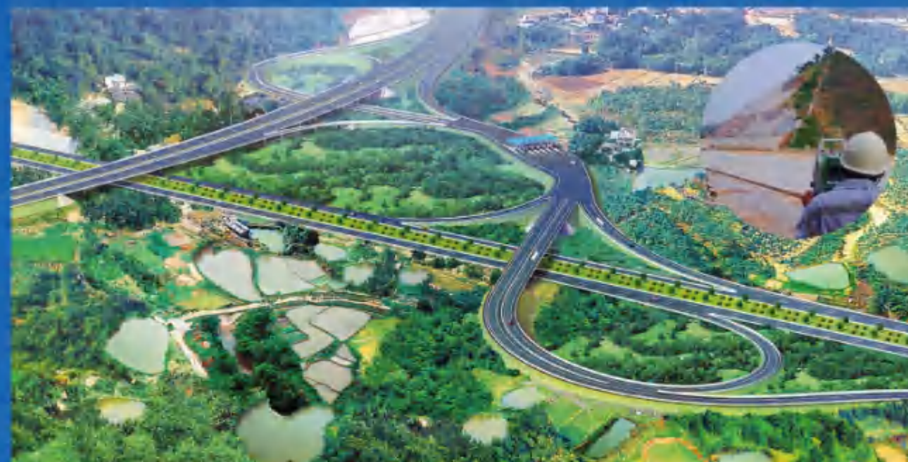
佛山市广明高速公路延长线高边坡工程监测 High slope engineering monitoring of extension line of Guangzhou-Gaoming Highway in Foshan
