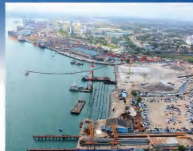
坦桑尼亚达港改扩建工程桩基PHC桩和灌注桩、高应变检测、低应变检测项目 PHC pile and cast-in-place pile, high strain detection and low strain detection items of Tanzanian Dagang reconstruction and expansion project
