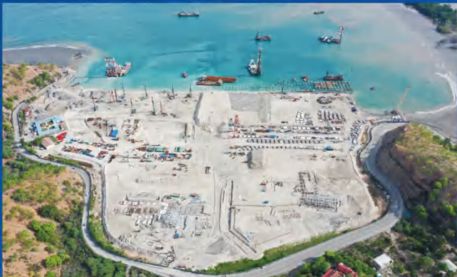
斯里兰卡汉班托塔港二期工程基坑边坡和围堰降排水及开挖过程中防渗墙的水平位移等监测 Monitoring of foundation pit slope and cofferdam drainage and horizontal displacement of cut-off wall during excavation of Hambantota Port Phase II project in Sri Lanka
