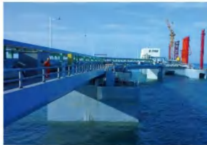
山东日照岚山港区耐久性监测与评估 Durability monitoring and assessment of Lanshan Port District in Rizhao, Shandong
