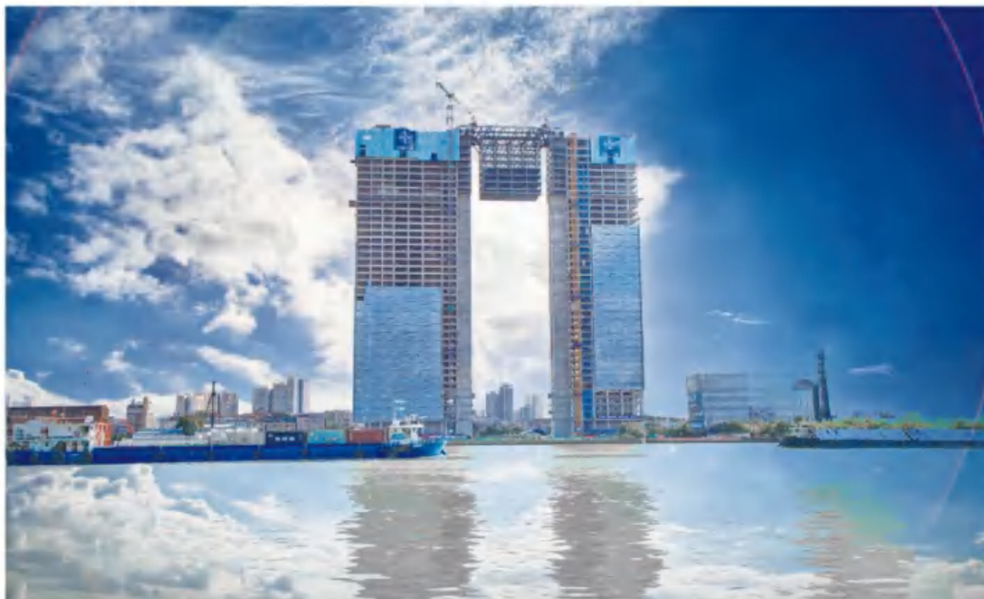
中交集团南方总部基地B区项目钢结构上、下连廊安装与提升施工监控项目 Construction monitoring project for installation and lifting of steel structure upper and lower corridor in Block B project of South headquarters base of CCCC
