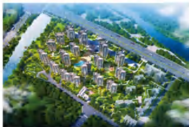
2012NJY-2地块（南珠）基坑监测 Monitoring of building excavation for Plot 2012NJY-2 in Nan sha district of Guangzhou
