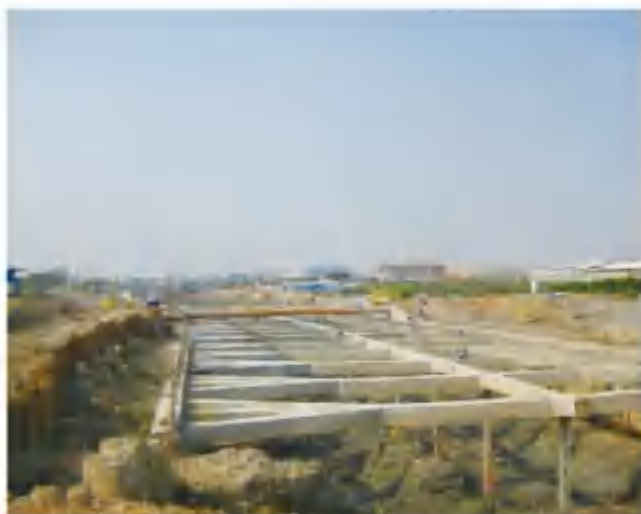
贵广铁路13标隧道（佛山隧道）基坑监测 Foundation pit monitoring of tunnel (Foshan Tunnel) of 13th Bid Section of Guiyang-Guangzhou Railway
