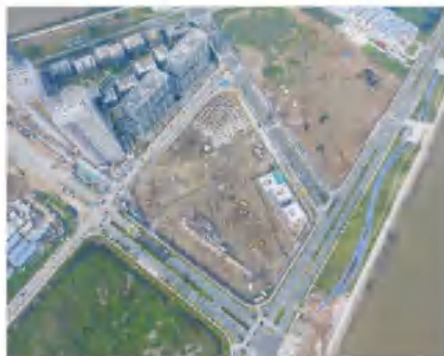
中交汇通中心基坑监测 Monitoring of building excavation for Huitong center of CCCC
