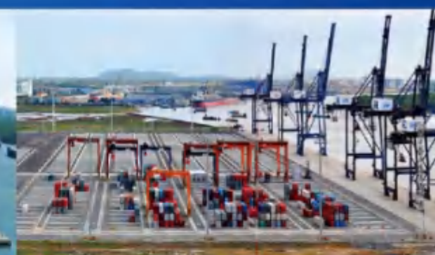
越南和黄西贡国际集装箱码头软基处理设计和咨询 Technical design and consultation of soft ground improvement for Saigon International Terminals, Vietnam
