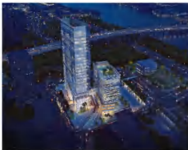
2014NJY-8地块（明珠湾开发大厦）基坑监测项目 Monitoring of building excavation for Plot 2014NJY-8 (Development Building of Ming zhu Bay) in Nan sha district of Guangzhou
