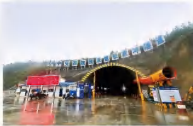
临武至连州高速张家冲隧道超前地质预报与监控量测 Advance geological prediction and monitoring measurement of Zhangjiachong tunnel in Linwu Lianzhou Expressway
