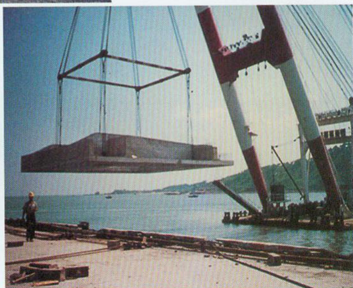
● “起九”吊船安装卸荷板
