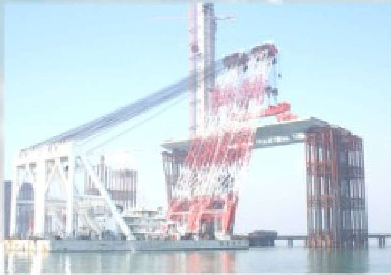
▲ 2600t “四航奋进”号吊装钢箱梁
