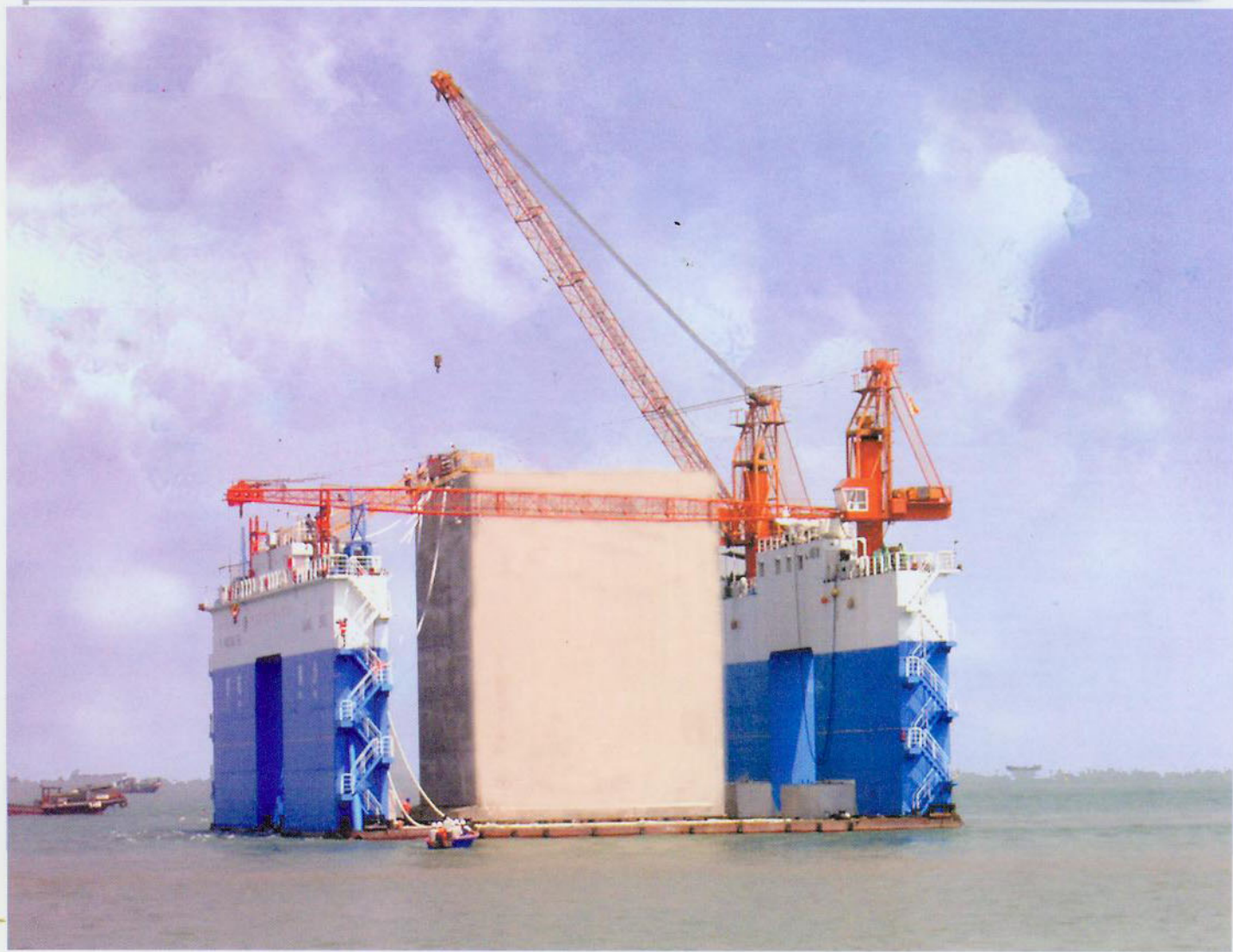
“四航南沙”号4100t浮船坞装运2212t大型沉箱
